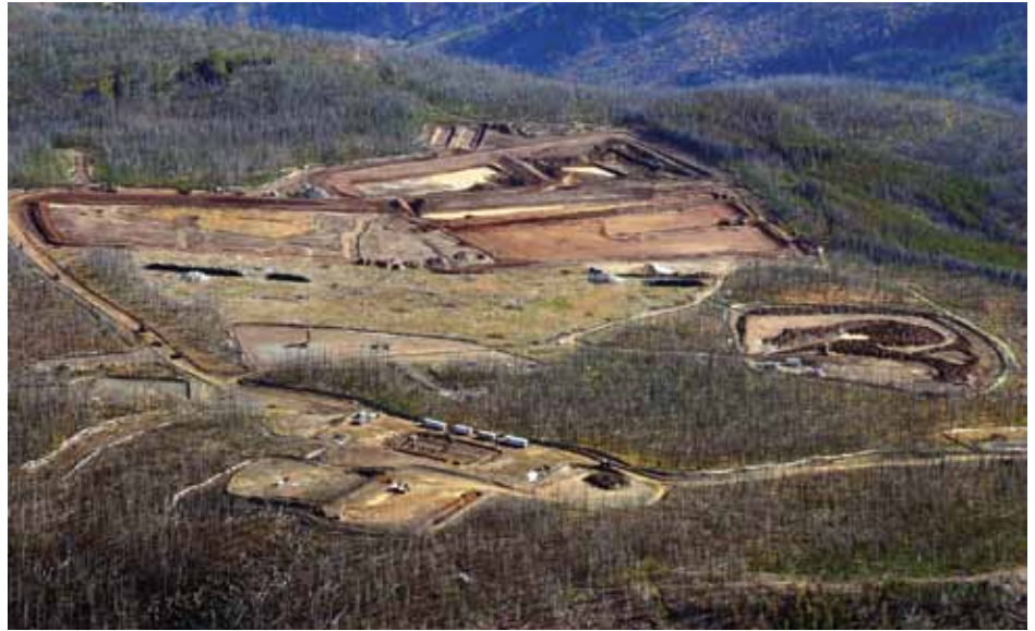
The Idaho Cobalt Project mill and concentrator pads, tailings waste storage facility and water management ponds' earthworks. Photo courtesy Formation Metals Inc.
