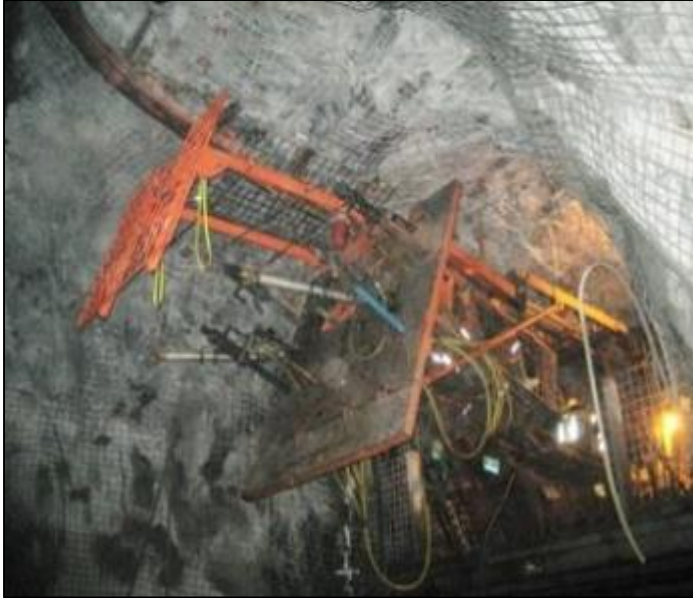
Alimak raise climbing equipment begins climbing up the first raise
