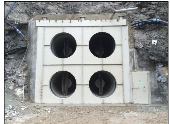
The exhaust fan installation at Wassa Underground
