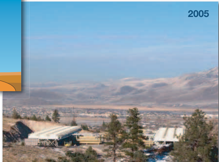
21 MW Burdette Geothermal Power Plant Nevada, USA
