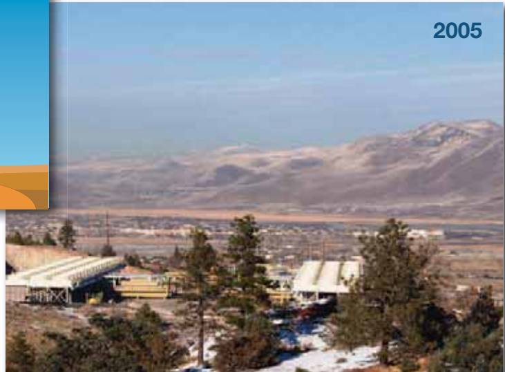
21 MW Burdette Geothermal Power Plant Nevada, USA
