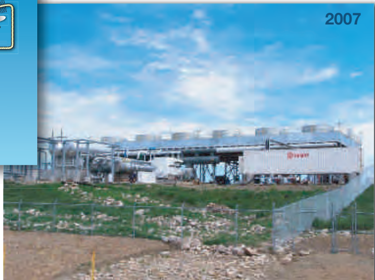
4x5.5 MW OREG at Basin Electric Cooperative Energy Generation Unit 1, North and South Dakota, USA
