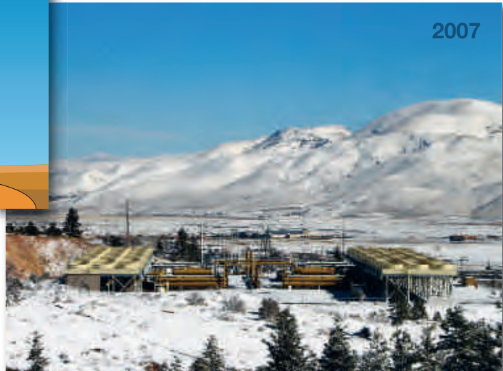
84 MW Steamboat Complex Nevada, USA
