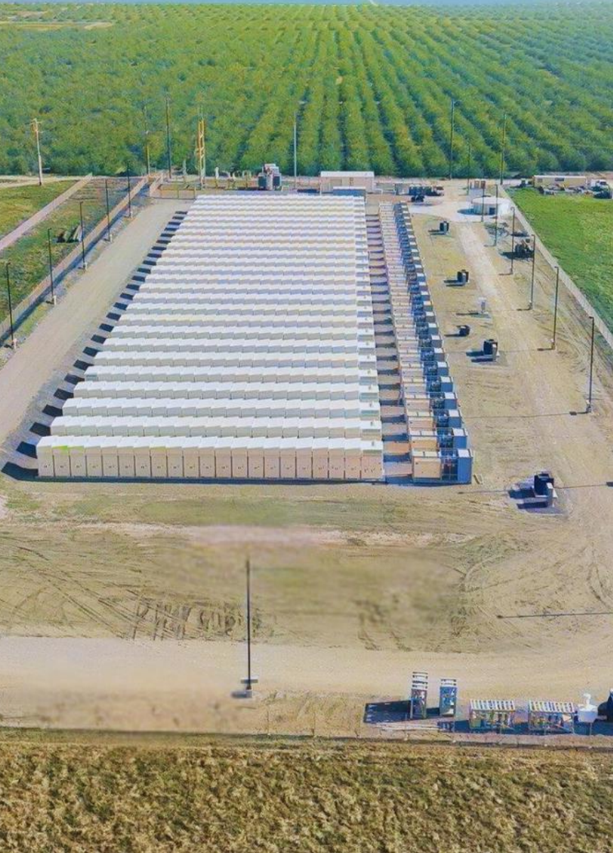
Bottleneck storage facility, CA, USA 80MW/320MWh
