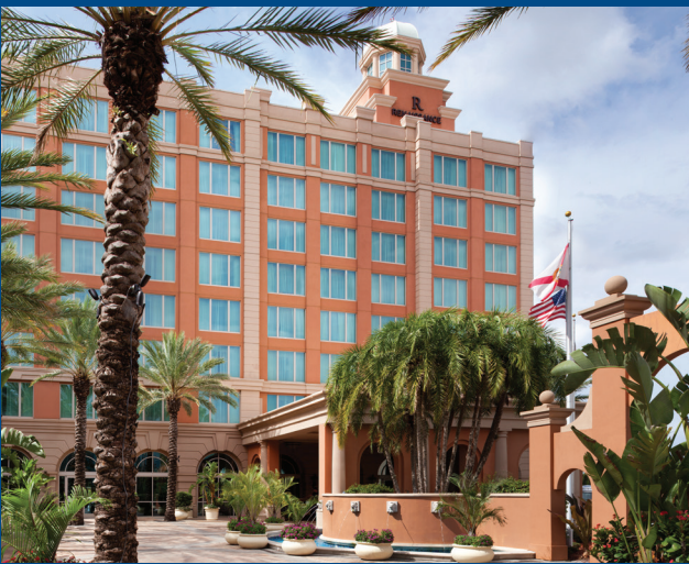
Renaissance Tampa Tampa, FL
