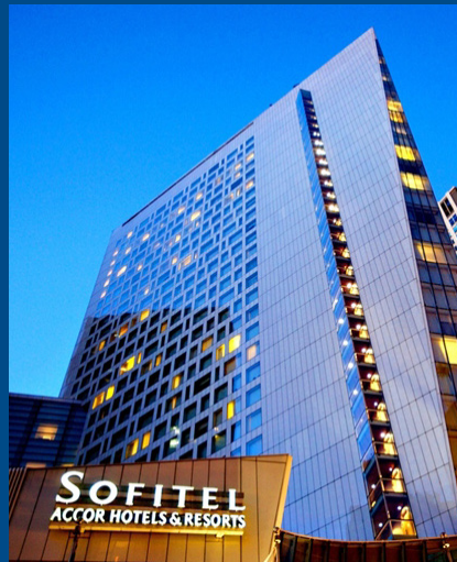
Sofitel Chicago Water Tower Chicago, IL
