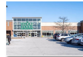
Elmhurst Crossing Chicago, IL
