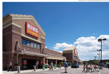
Centennial Shopping Center Denver, CO
