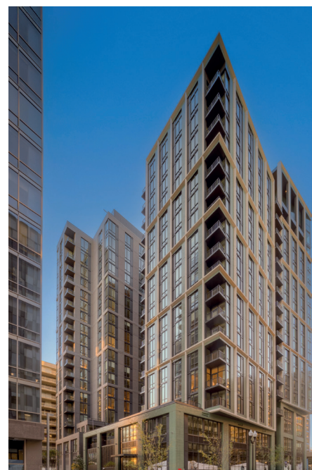
2001 South Bell Street (under construction multifamily asset)
