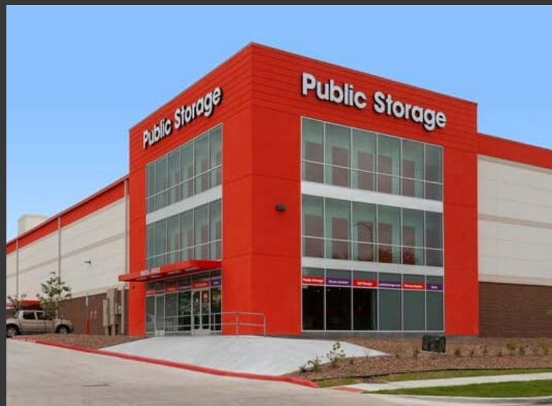
Flood Resilient Redevelopment Houston, TX
