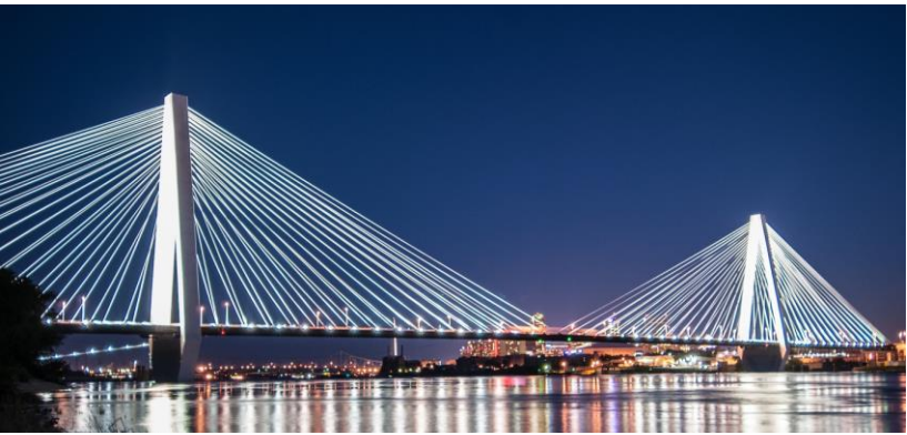
W&W | AFCO Steel | Oklahoma City, OK Fabricator and erector of structural steel for commercial, manufacturing and transportation infrastructure projects.
