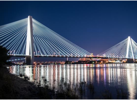
W&W | AFCO Steel | Oklahoma City, OK Fabricator and erector of structural steel for commercial, manufacturing and transportation infrastructure projects.
