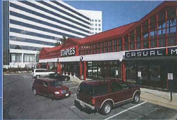
11503 Rockville Pike, Rockville, Maryland
