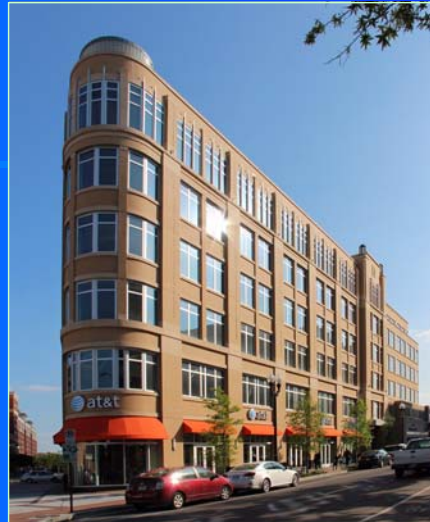
North Block Office Building
