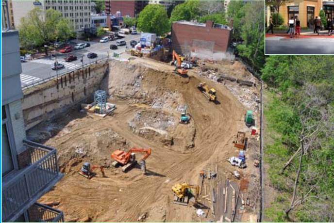
Construction Progress Photo, May 8, 2014
