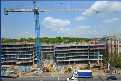
Progress Photo, May 6, 2015
