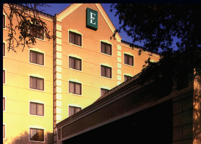
Embassy Suites Dallas - Near the Galleria Dallas, Texas
