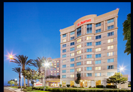
Freemont Marriott Silicon Valley Freemont, California
