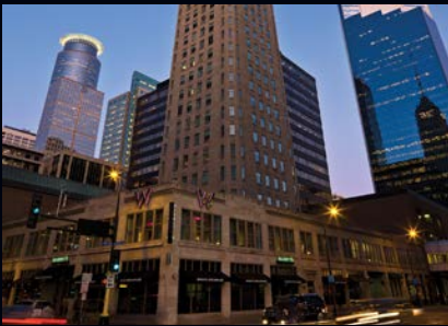
W Minneapolis - The Foshay Minneapolis, Minnesota
